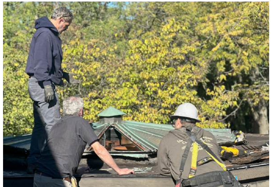
Restoring the skylight over the Library in Wright's Studio
